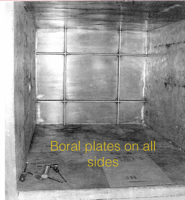
The end wall consists of 2-in. x 3/8-in. webbing, 1-in. thick sheet, and 1/4-in. thick pool liner, all 6061 aluminum.
